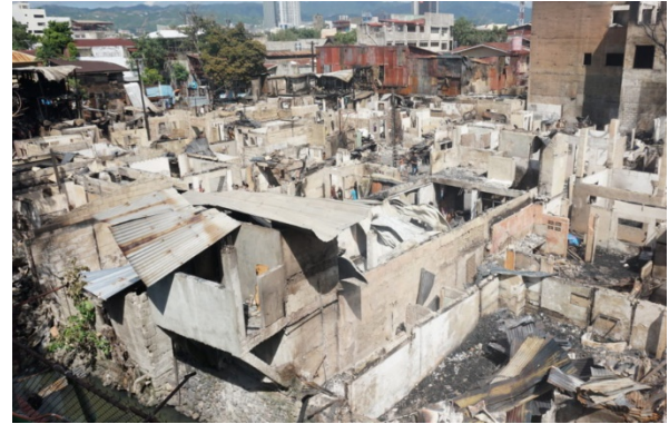
Figure 5. 11: Aerial view after the fire
