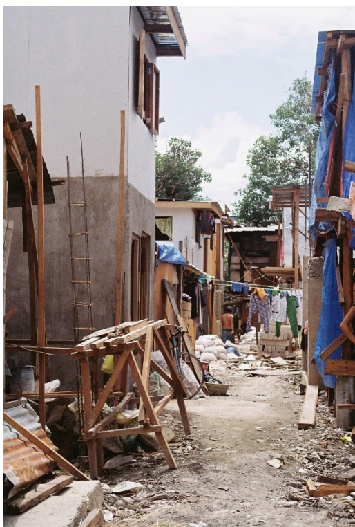
Figure 5. 19: Self-Build Reconstruction in Sitio Panting (Source: Liu Ly Chan)
