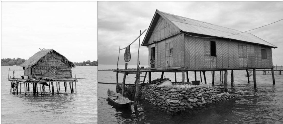
Figure 6. 1: Water stilt house (left: temporary house, right: permanent house)
