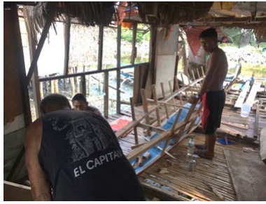
Figure 6. 58: Site A Ship making work (Source: Wakana Katsura)
